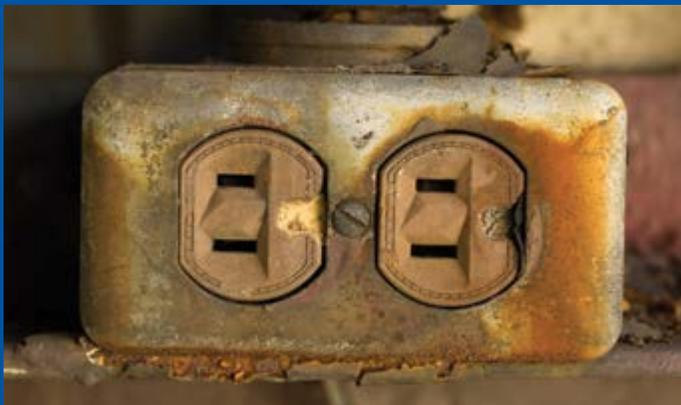
**3.** You have no three-prong outlets. Some older homes were built with two-prong outlets only. Sure, you can buy cheap three-into-two adapters at the hardware store, but it may be that your electrical wiring is not fully grounded. For safety sake you are better off installing some three-prong outlets for your microwave, refrigerator and other heavy appliances that require them.
