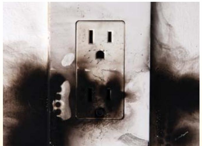
**Open or damaged junction boxes.** A junction box houses the splices where wires are connected, and we occasionally find them with the cover damaged or missing.
